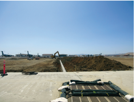
Storm drain installation of concrete in front of paver; End product of 17.5 inch thick paving.
